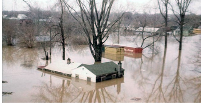
Recent Floods in Michigan, Over 18,000 Homes Flooded, Photo by NOAA
