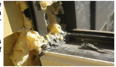
Foam Plugging Window Weep
